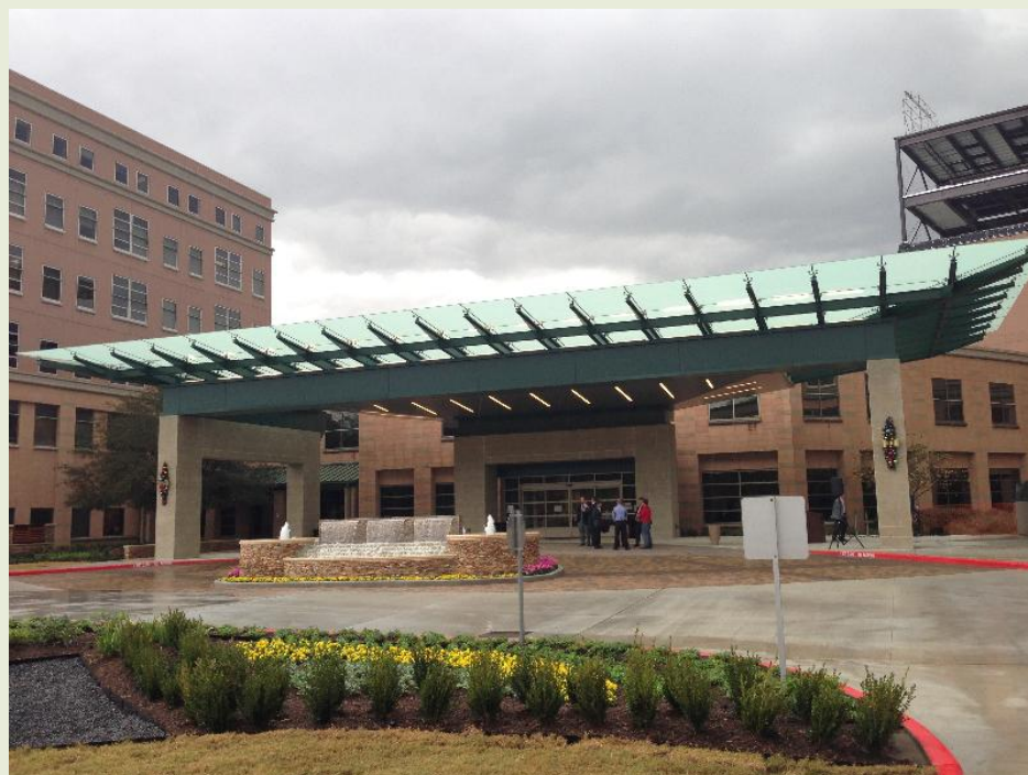
St. Luke's Woodland's new entry canopy
